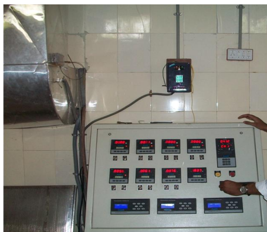
Fig 7. Power Control Unit of Solar Dryer
